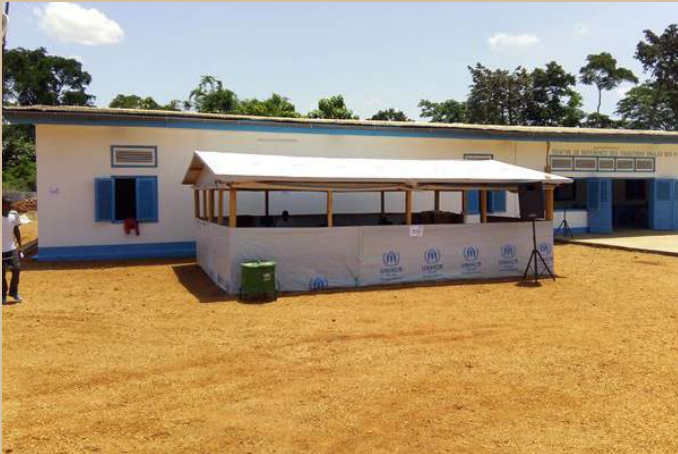
Moungoumba transit center after rehabilitation by AIRD CAR Program
