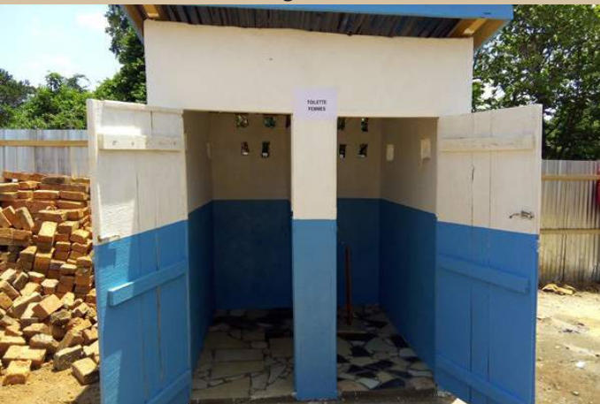
Toilets constructed by CAR Program at the transit centre in Moungoumba
