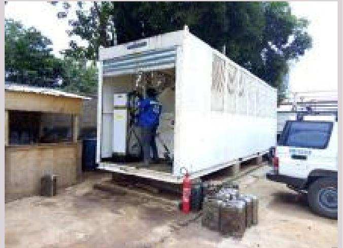
*Fuel station in Bangui CAR. Fuel stations used in CAR are made of a movable container that includes a fuel dispensing pump and fuel storage tank*
