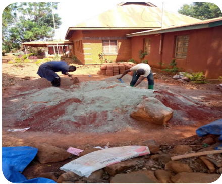
Mixing soil and cement for brick fabrication (left), putting up the walls (centre) and a completed registration building at Nduta camp (right).
