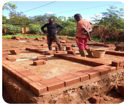
Mixing soil and cement for brick fabrication (left), putting up the walls (centre) and a completed registration building at Nduta camp (right).
