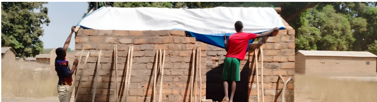
Odile's house is temporarily sheltered by a tarpaulin, one of the essential materials provided by AIRD as part of their emergency response efforts.
